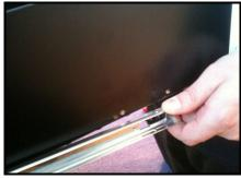
Position the metal tabs on each runner in line with the cut outs in the drawer
