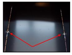
The drawer is held in place by a small metal tab on each of the runners which slot into small cut outs in the base of the drawer.
