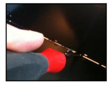
Slot the metal tabs on the runners back into the cut outs. *You may need to use a flat head screwdriver to help lever back in.*
